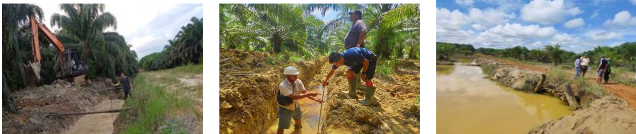
Figure 6: Monitoring fields during the embankment project
